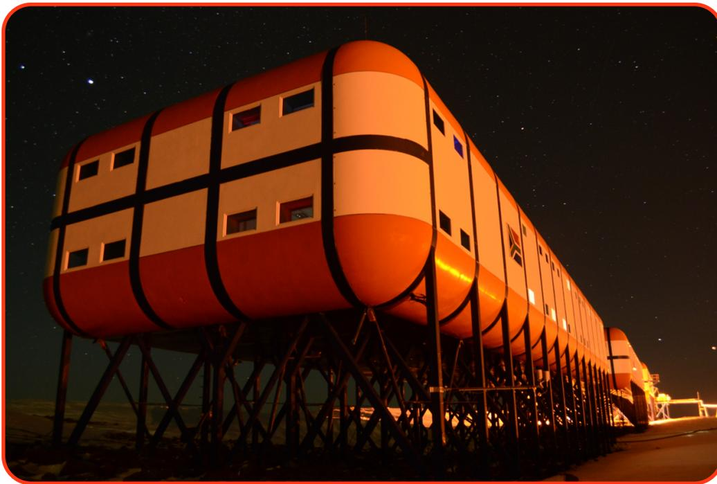
composite nature with steel foundations and frames and with fibreglass, aluminium and foam panels inserted into the frames. The rounded edges are designed specifically to reduce wind drag, which was
